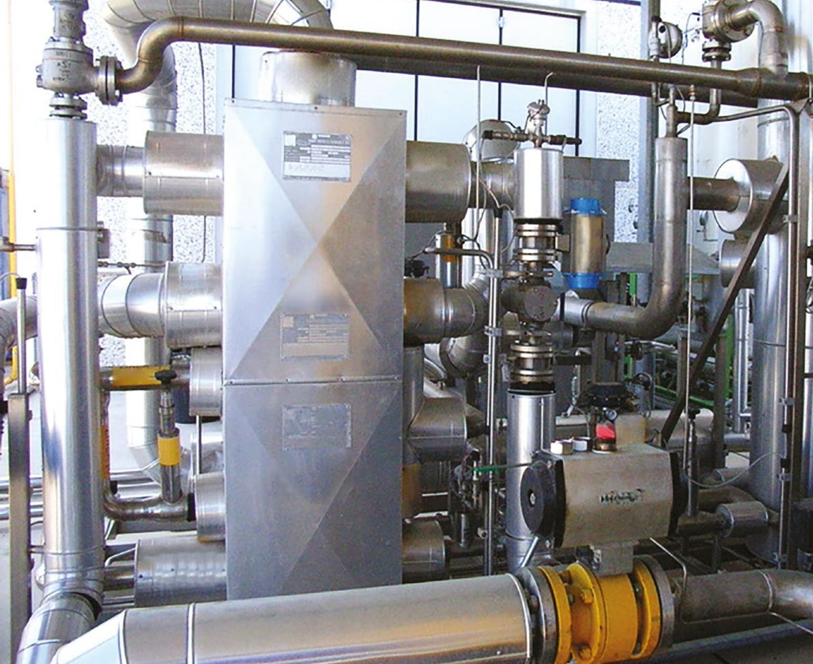
Technology developed by S.TRa.Te.G.I.E. S.r.l. based on patented optimization of a modified Linde cycle.
